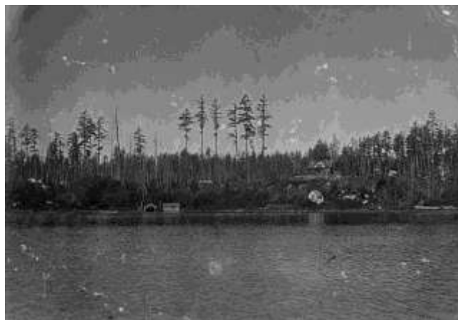
Lake, pump house(?) to left and house to right
